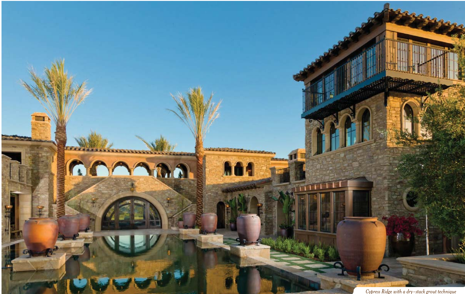
Cliffstone with a dry-stack grout technique
