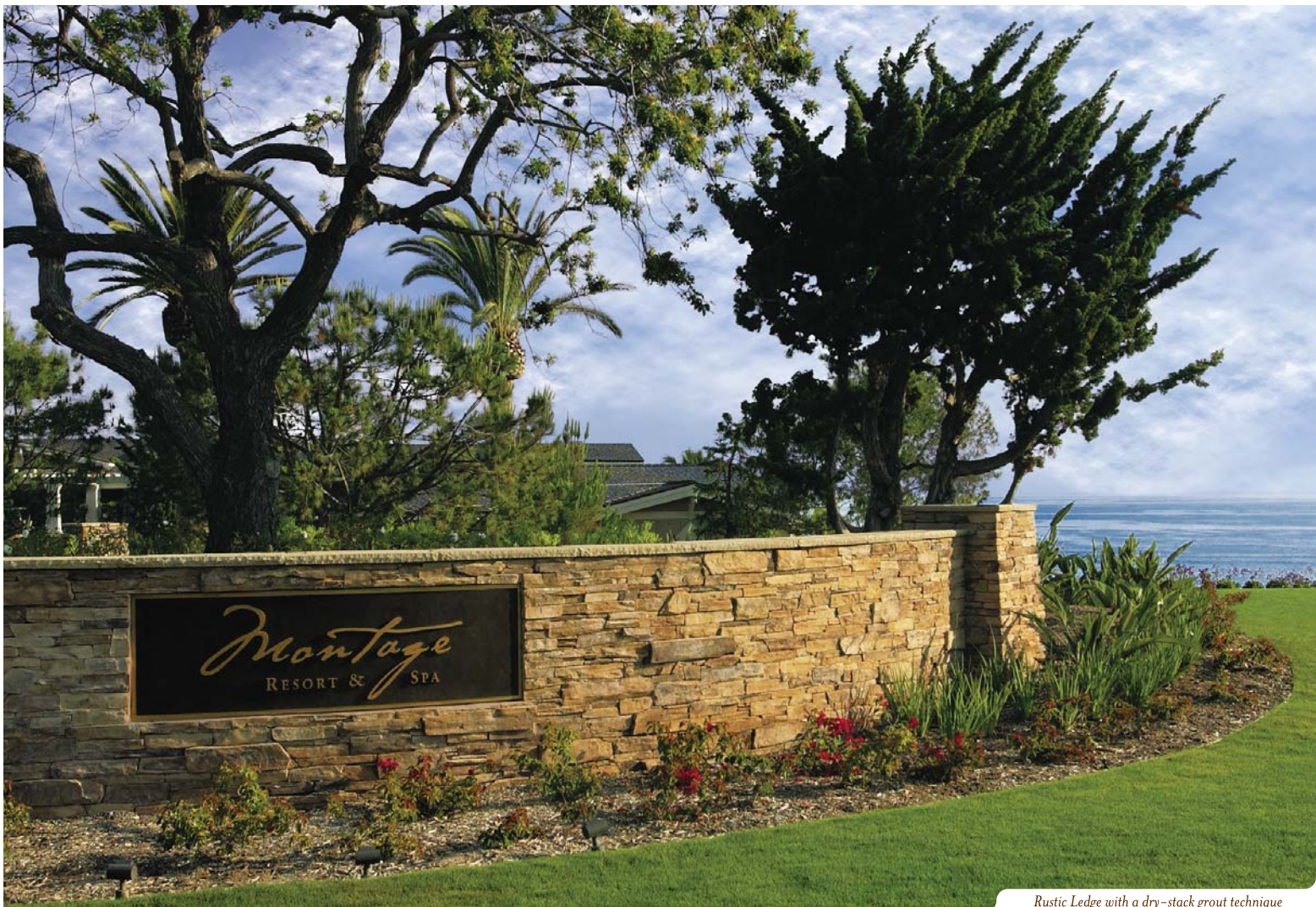
Rustic Ledge with a dry-stack grout technique
